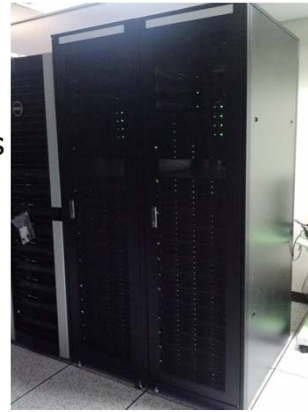
500TB storage servers
